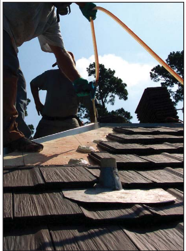
POLYFOAM BEING APPLIED TO DECK DURING INSTALLATION OF US TILE.
