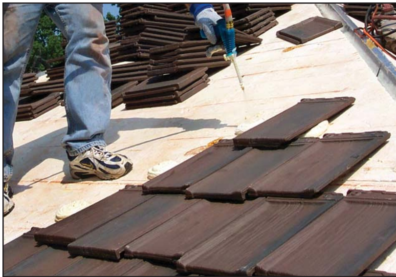
POLYFOAM BEING APPLIED TO DECK DURING INSTALLATION OF US TILE.
